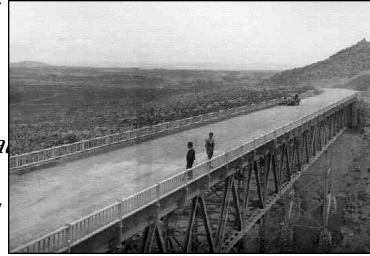
Figure 19. The bridge spanning Dead Indian Canyon along the original East Approach Road from Cameron, ca. 1935. Today's approach road from Cannon was rebuilt to the north (left) of this bridge in the 1960s, although the bridge still stands. GRCA 2920.
