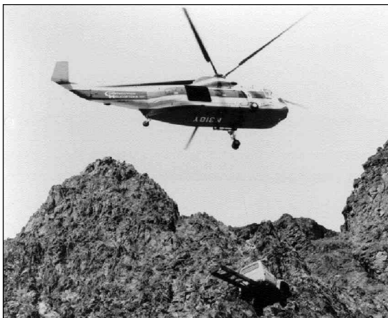
Figure 43.A Sikorsky S-61 carrying a truck down to Phantom Ranch to facilitate construction of the trans-canyon pipeline May 1968. GRCA 5208.
