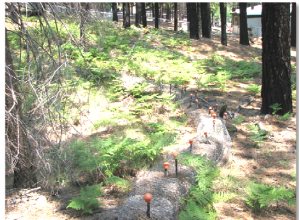
Image 5-7: Post construction of hay bale structures above Zimmerman School, Mt. Lemmon, 2007.
