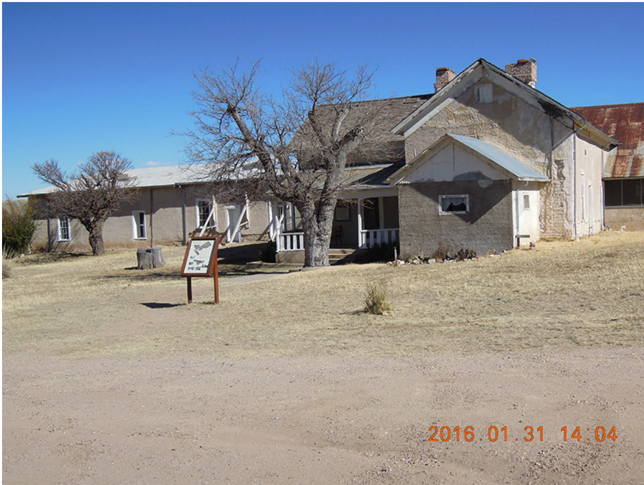
Figure 9. Main Ranch House with Original Ranch House (left) and Victorian and Children's Additions (right) Facing East. Gina Chorover, 2016.
