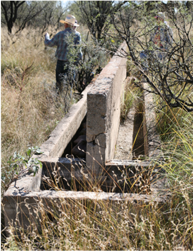
Figure 49. Double-Sided Concrete Watering Trough at Orchard. Robin Pinto, 2016.
