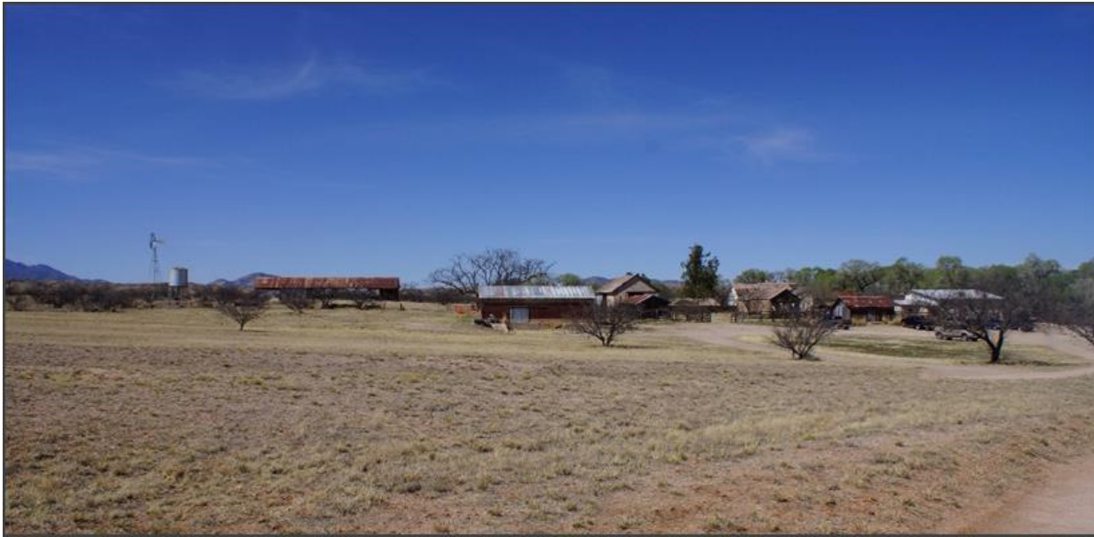
Figure 7. View of Main Empire Ranch House Area Facing West. Taira Newman, 2016.
