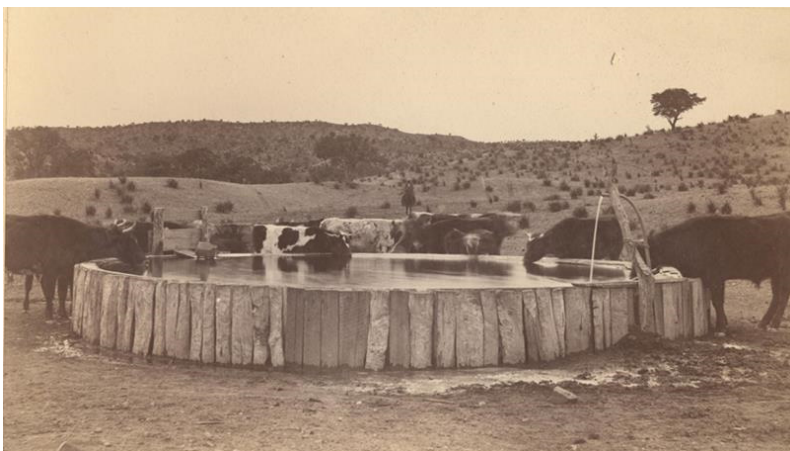
Figure 48. Edward Vail's VR Ranch Water Tank. Circa 1890s. Courtesy of the Empire Ranch Foundation (A448-1A).
