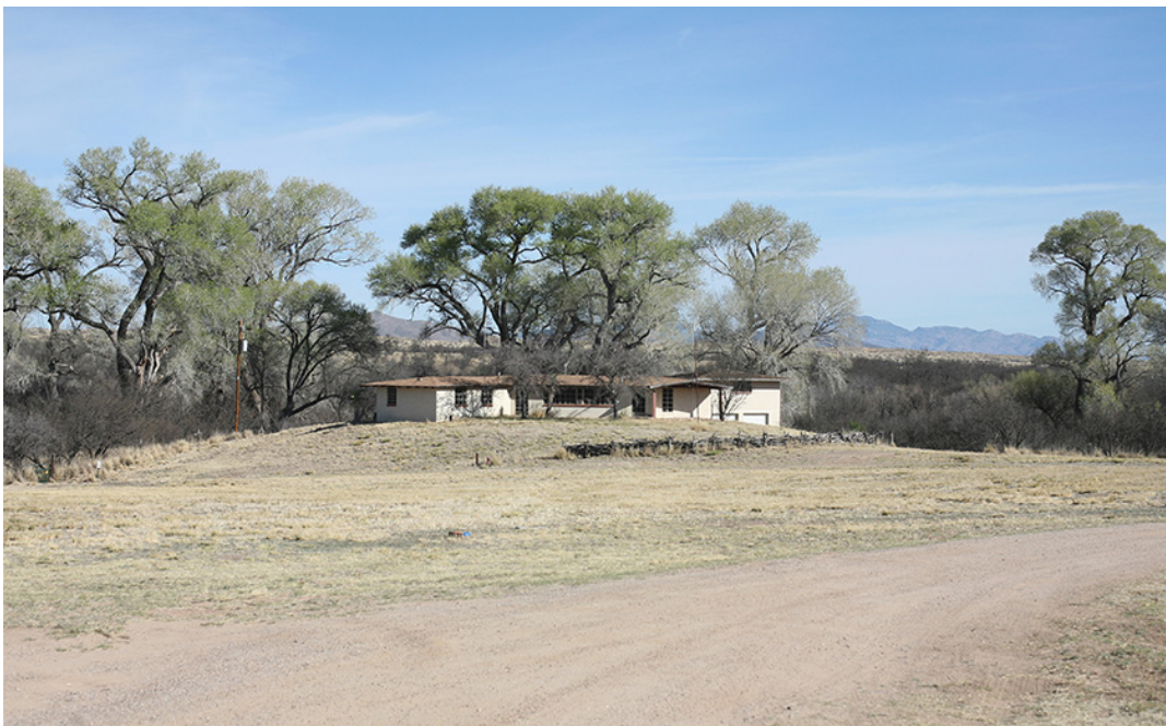
Figure 22. The New Ranch (or Pancho's) House, Facing North, with Empire Gulch and Cottonwoods in Rear. Robin Pinto, 2016.
