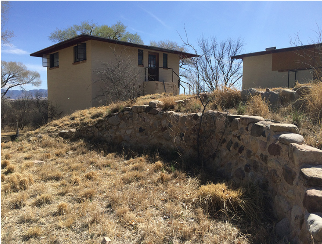
Figure 23. Stone Retaining Wall and Garage on North Side of New Ranch House. Kathryn McKinney, 2016.
