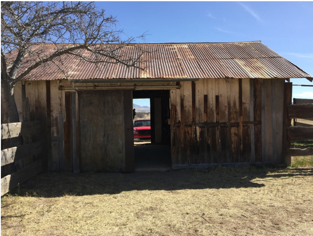
Figure 28. Exterior of Tack Room, Facing East. Abrar Alkadi, 2016.
