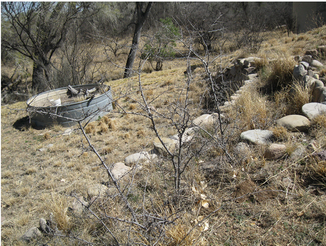
Figure 52. Water Tank or Pool, North Side of the New Ranch House. Jessica Estrada, 2016.
