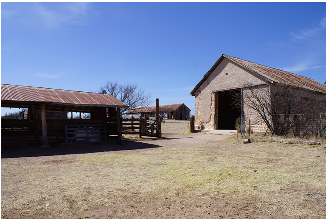
Figure 30. Adobe Haybarn, Right; Covered Feed Trough with Corrals, Left; South Barn in Background. View Looking Southwest. Taira Newman, 2016.
