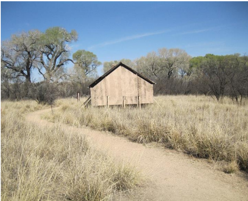
Figure 35. Restored South Façade of the Hired Man's House. Jessica Estrada, 2016.
