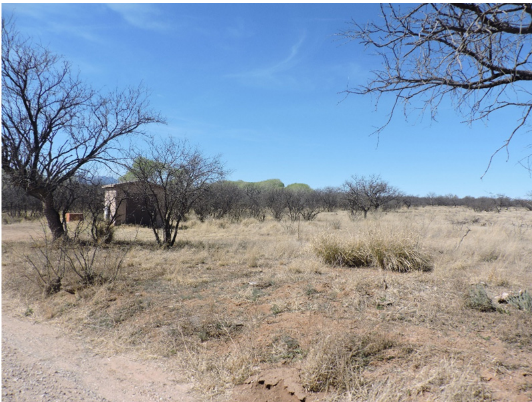
Figure 45. Pump House, North of Empire Gulch. View looking West. Nicole Lavelly, 2016.
