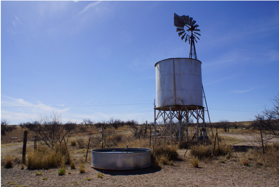
Figure 32. Modern Cattle Water Trough, Water Tank and Windmill. View looking South. Taira Newman, 2016.
