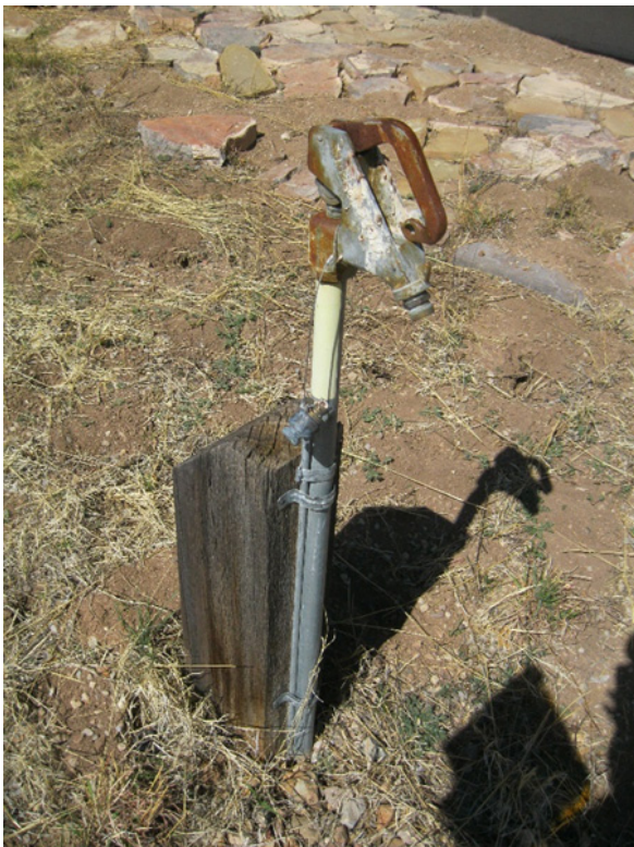
Figure 24. Water Spigot South Side of the New Ranch House. Jessica Estrada, 2016.
