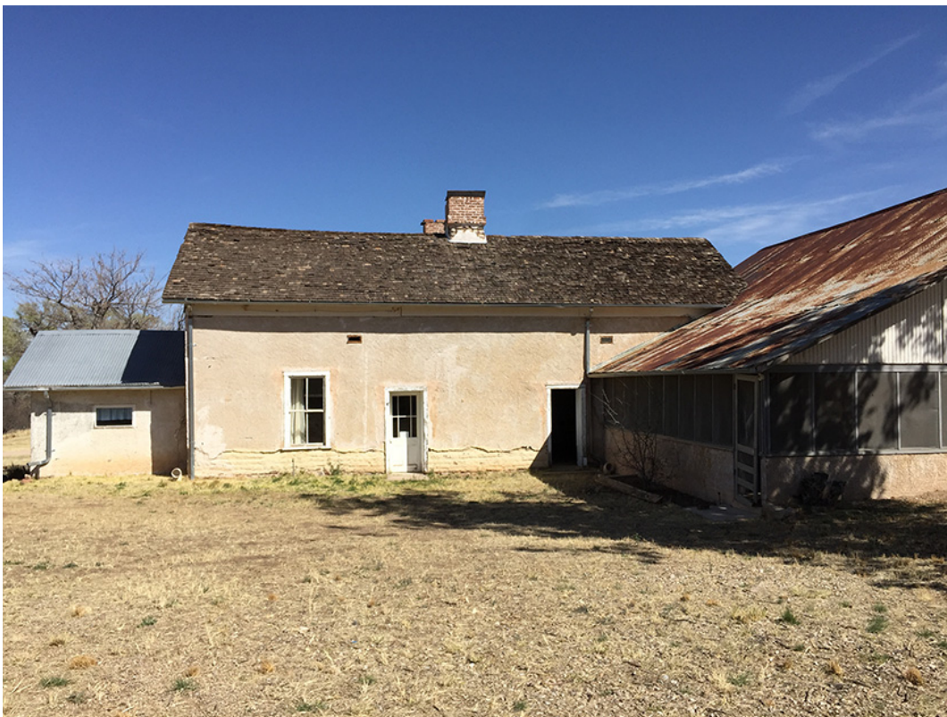
Figure 14. South Yard with Children's Addition and Screened-In Porch Right. View Looking North. Abrar Alkadi, 2016.
