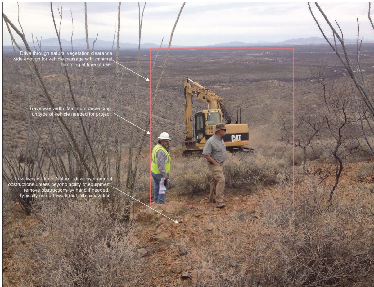
Figure E-5. Typical Overland Access Route: Narrow, very low volume, two track vehicle access route used for authorized administrative purposes for maintenance, operation, repair or replacement of existing facilities or improvements, or special projects that require vehicle access to transport tools, materials or supplies that can-not be transported by non-motorized means. These routes include existing routes previously constructed, but are not intended to accommodate regular on-going vehicle traffic. These routes will be allowed to reclaim naturally after each use, and restoration treatments may be applied if disturbance is likely to attract more use, or have a persistent impacts.
