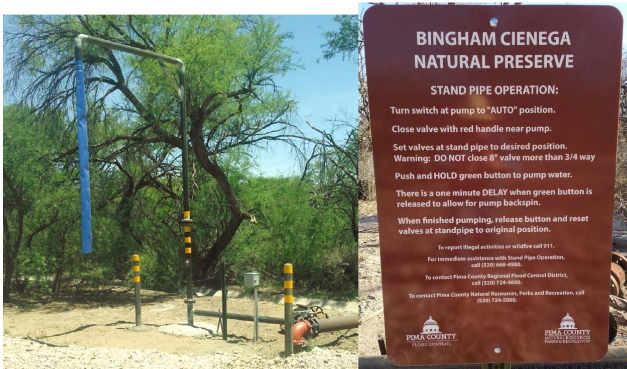
Figure 10. All-weather water station installed in 2017 and operational signage installed in 2018 at the Bingham Cienega Natural Preserve.
