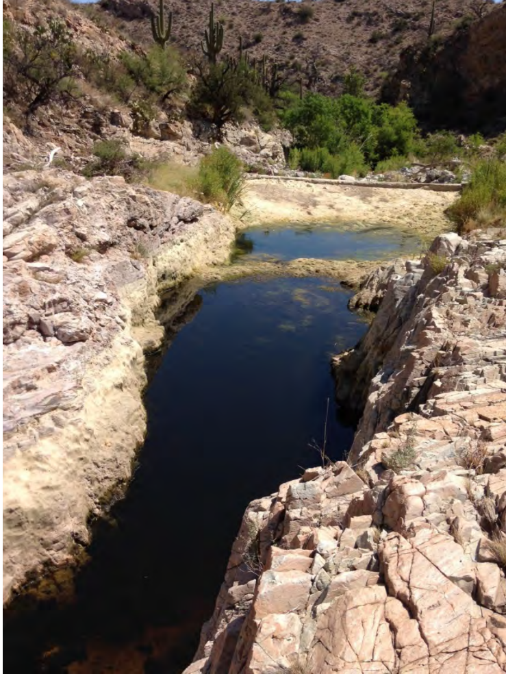
Figure 23. Large pool in Bullock Canyon, with cement dam visible in the background.
