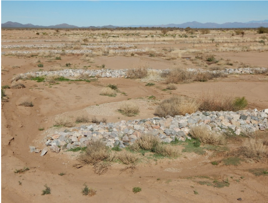
Figure 19. NAWA rock structures after maintenance treatments, with water erosion flow paths evident around the left side of the structures.
