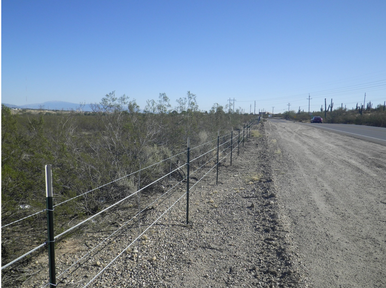
Figure 21. OHV-resistant fencing installed during 2019 at the District’s Ina Preserve, along the Santa Cruz River to prevent ongoing and illegal incursions into the area. Note the two heavy cut-resistant cables.
