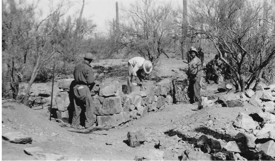
Figure 15. Building with stone, SAGU257, Series 4, Box 4, WACC.
