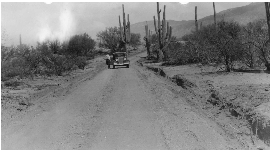
Figure 26. “New road recently graded in Saguaro National Monument. Note narrow roadbed, high crown, bad unsightly ditches—no sloping.” SAGU257, Box 4, Folder 17, WACC.
