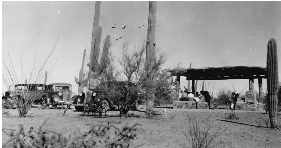
Figure 16. Saguaro rib veneer on concrete posts, stone foundations, SAGU257, Series 4, Box 4, WACC.
