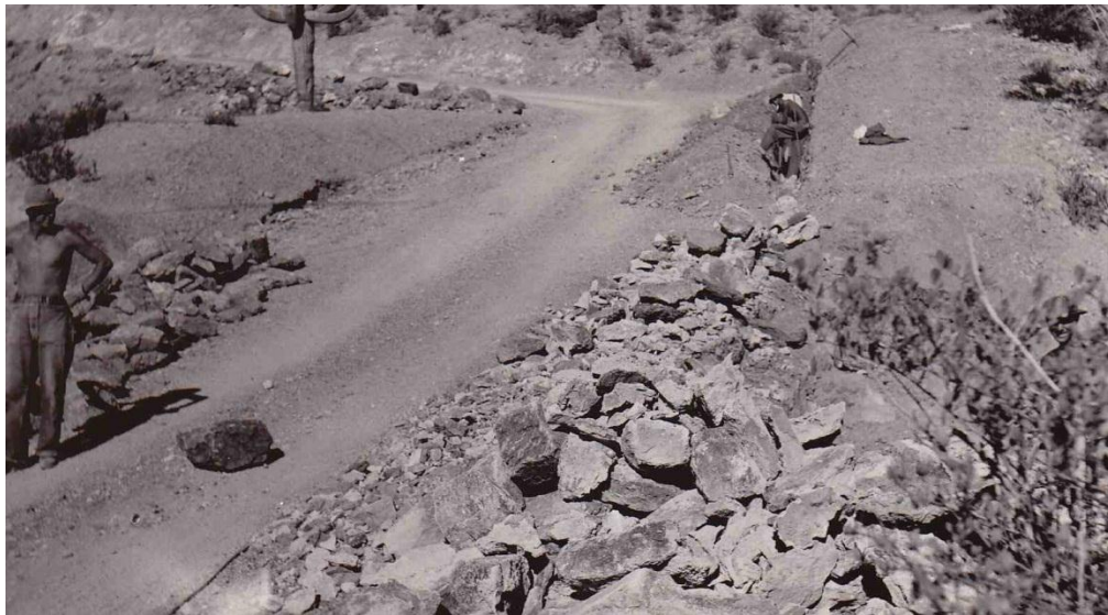
Figure 10. "Before sloping & planting of bank slope, near a mountain grade culvert in the Gates Pass mountain area." SAGU257, Box 3, Folder 20, WACC.
