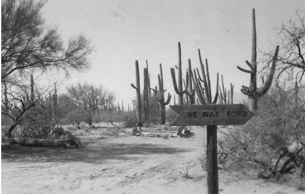
Figure 28. Working to define the loop road in the 1930s, SAGU 257, Series 4, Box 4, WACC.
